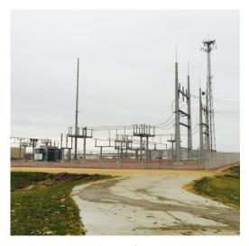
Northport substation located at site (opposite the southern edge of site) is unused with 27 MVA capacity, looped from the Penelope substation (1.5 mi NW) and Johnson substation (1 mi SE) of site
